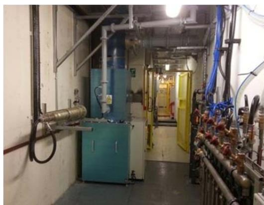
*Figure 3: First triode amplifier installed in the MICE hall*
