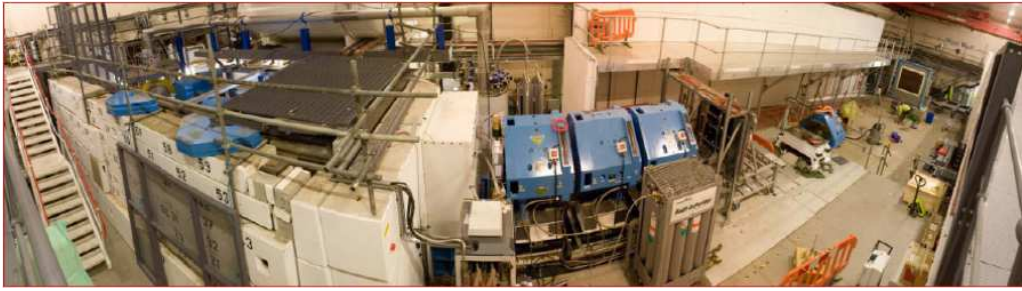
Figure 4: Fish-eye view of the MICE installation
